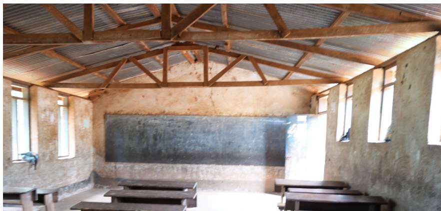
Figure 4.4. A Tanzanian classroom, showing the structure of the rafters and roof
