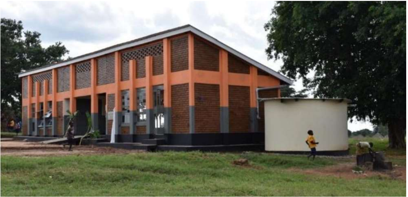
Kumel School building, Uganda, constructed using interlocking stabilised soil blocks with hit-and-miss ventilation openings at the top courses and rainwater harvested in an ISSB* constructed tank [Haileybury Youth Trust designed by RFF].
